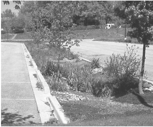
Figure 3. Photo of parking lot with established landscape islands for infiltration of runoff. (Courtesy of Prince George's County, MD)
