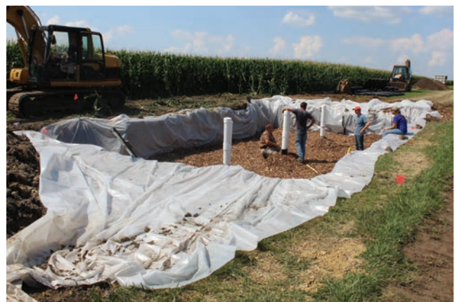
Fig. 11.5. Construction of a denitrifying woodchip bioreactor at the University of Illinois Department of Crop Sciences Northwest Research and Education Center near Monmouth, Illinois (image: J. Chandrasoma/UIUC).
