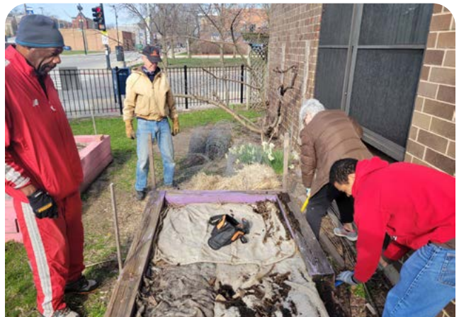
Repairing raised beds at community outreach organization.
