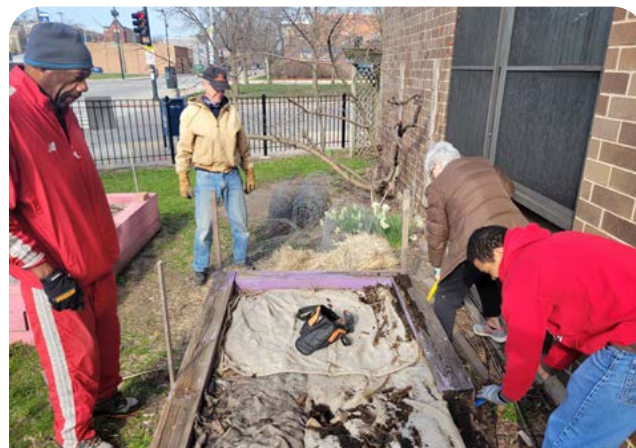
Repairing raised beds at community outreach organization.
