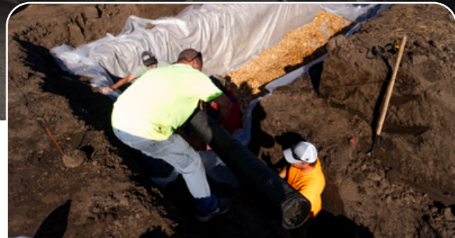
Haverback organized a bioreactor installation demonstration to showcase an effective strategy for nutrient loss reduction.
