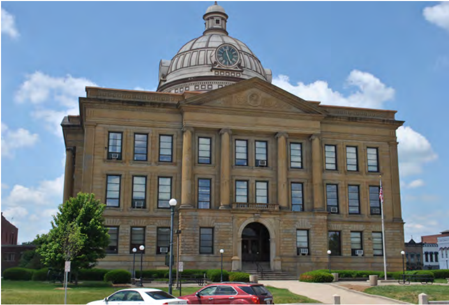
Figure 19: Court House in Downtown Lincoln, IL
