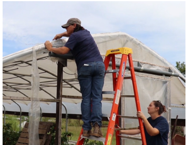
Local Foods and Small Farms Educators Katie Bell and Bronwyn Aly replace the walls of the demonstration high tunnel.
