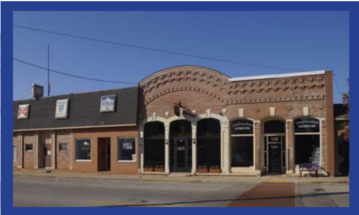
The removal of the modern storefront to reveal the historic brickwork during the rehabilitation of this west facade reveals important unique details of the historic facade.
