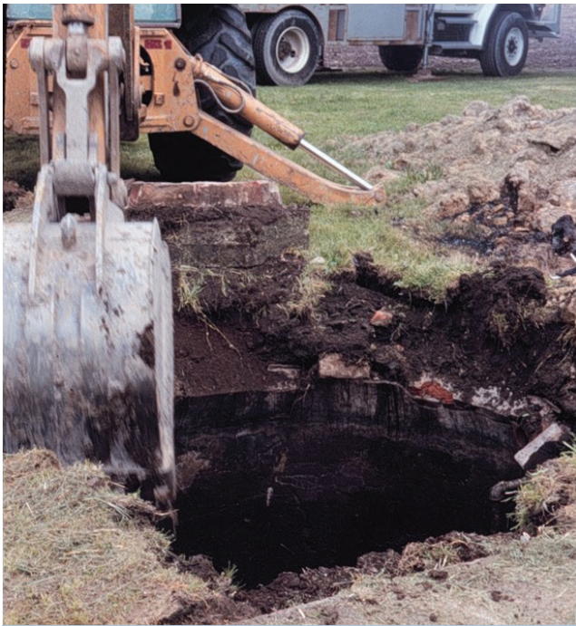
Fig. 7.1. Sealing an abandoned well in Illinois (Credit: G. Czapar, UIUC)
